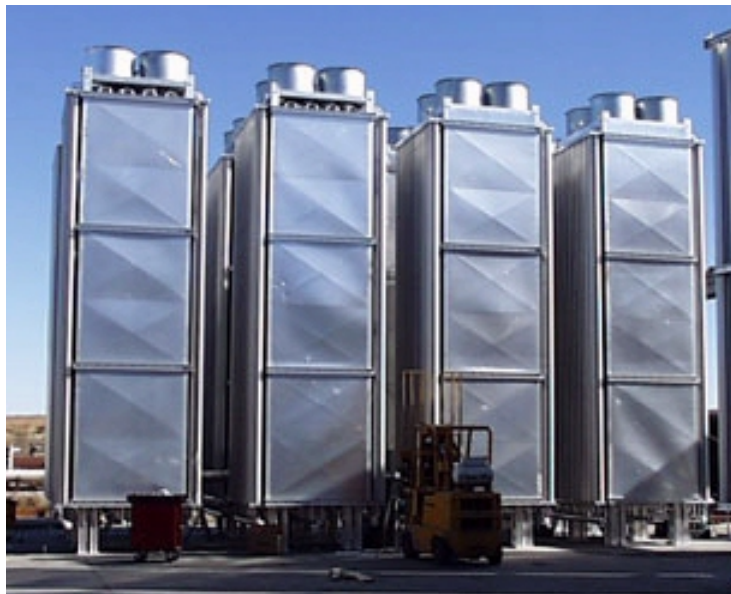
Figure 11: Direct Forced Draft Ambient Air Vaporizers - with shrouds
