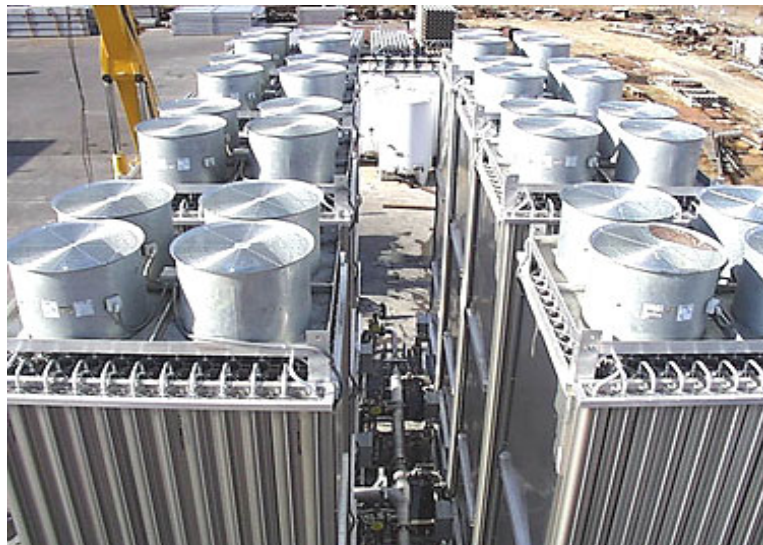
Figure 10: Direct Forced Draft Ambient Air Vaporizers - without shrouds
