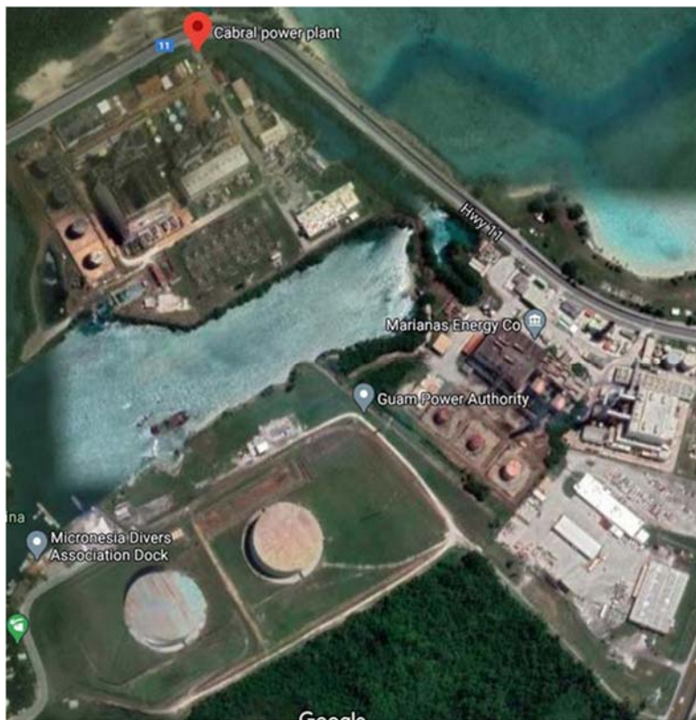
Figure 16-7. GPA Bulk Fuel Storage Facility (Delivery Pump Station located adjacent to the site office)
