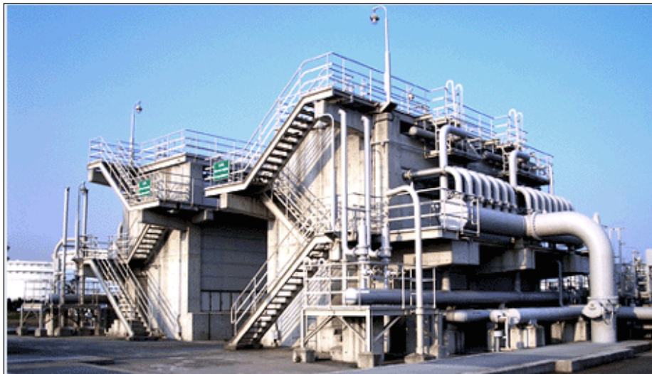
Figure 4: Typical 2 each Open Rack Vaporization (ORV) Arrangement
